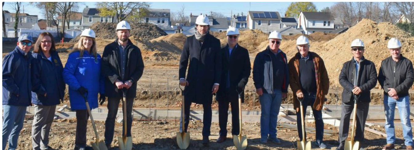
Town of Stratford officials and members of the development team for The Village of Stratford at a recent groundbreaking. Photo courtesy of Mayor Laura Hoydick
