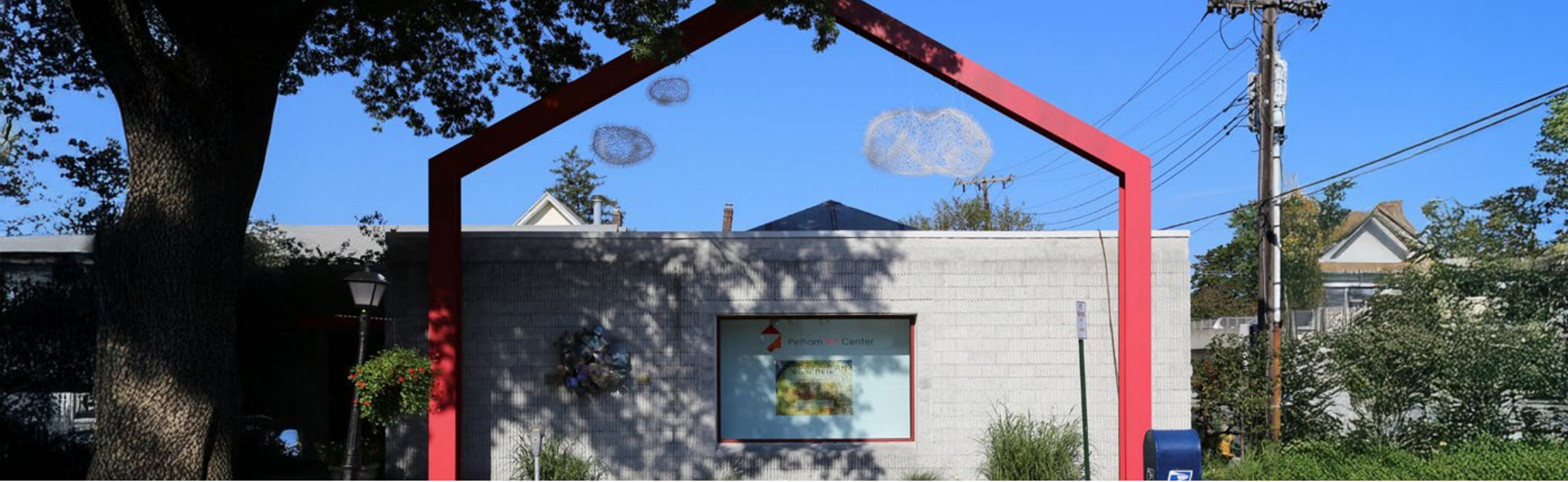
The Pelham Art Center, on the site of a former Citgo gas station, recently underwent a $500,000 revamp as part of an ongoing capital campaign. The artwork in the window is Sui Park's "Cloud Nine." Photographs courtesy Pelham Art Center.
