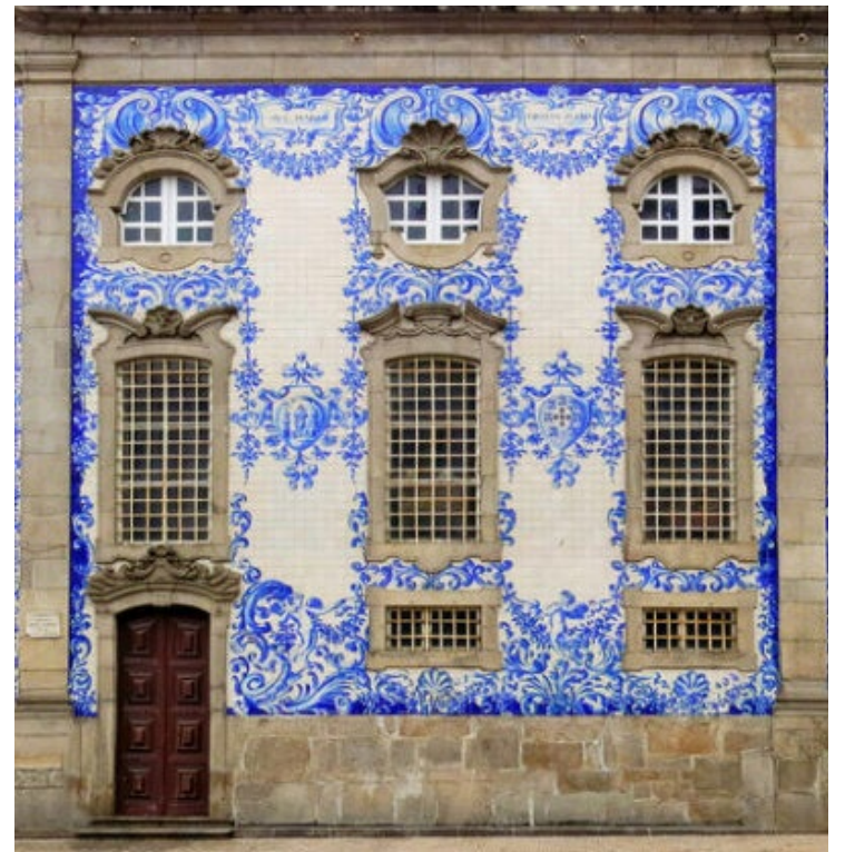
The façade of this tony house in Porto, Portugal, is covered with antique tiles (azulejo), painted ceramics that are a major part of Portuguese architecture.
