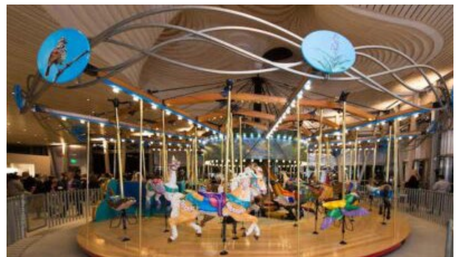
At Mill River Park, nature meets culture in the forms of free, year-round programming and in such modern, sustainable structures as the Brownstein | Selkowitz Carousel Pavilion.
