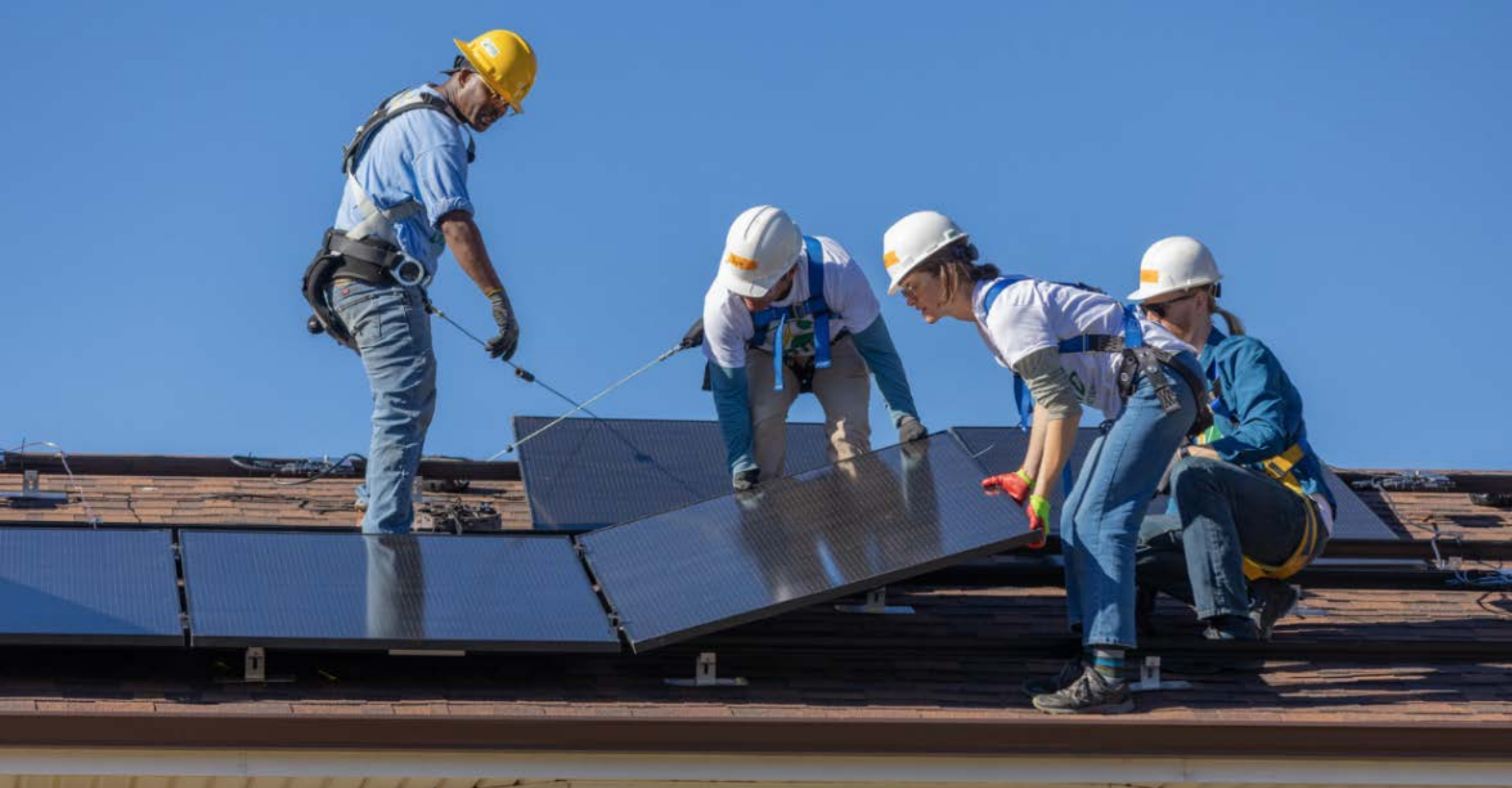
Installing solar cells on house under construction.
