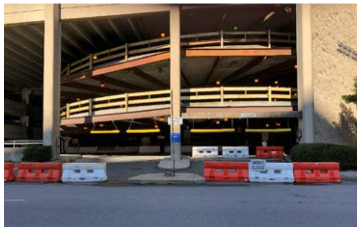
Closed entrance at Lexington-Grove West Parking Structure.
