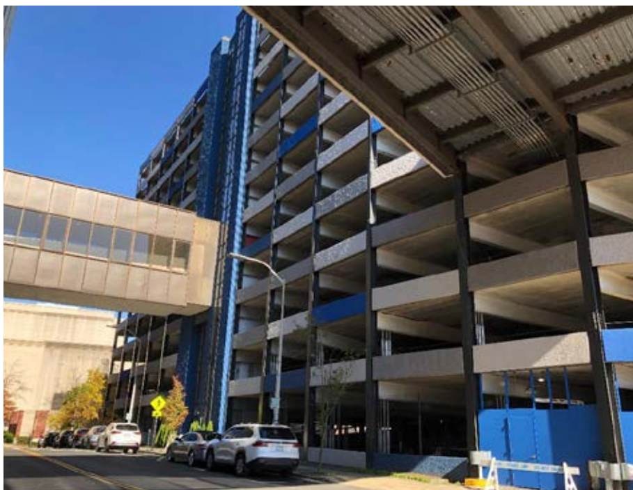
50 Hale Ave. garage. Photos by Peter Katz.
