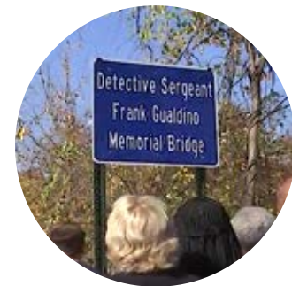
A Tuckahoe Road overpass bridge was dedicated to the memory of Yonkers Det. Sgt. Frank Gualdino.
