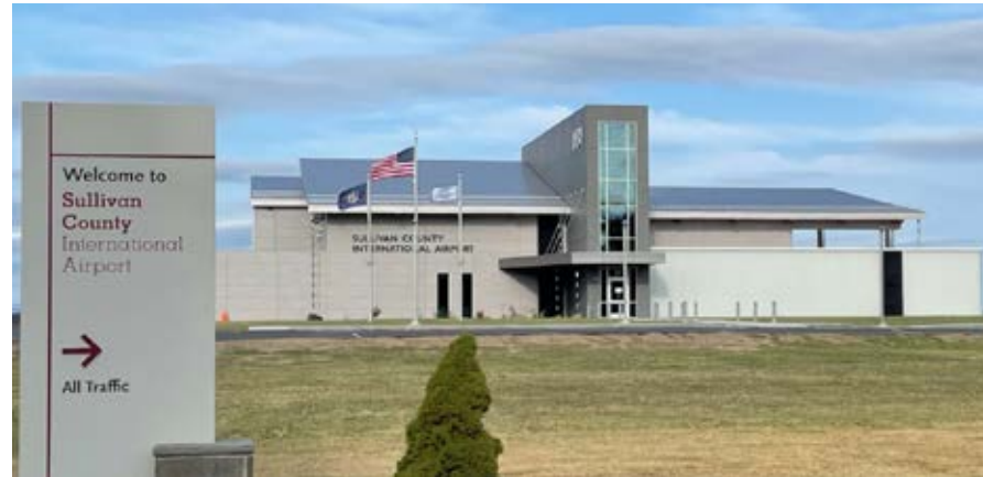
New terminal building at Sullivan County's airport.
