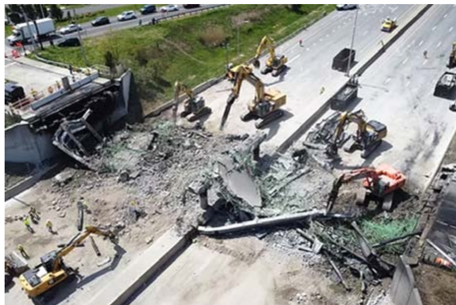
Demolishing the I-95 bridge at Norwalk.
