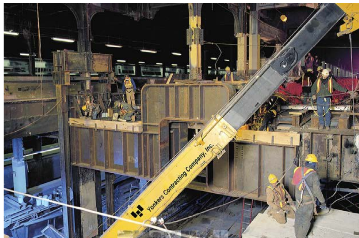
Yonkers Contracting crew at work at Grand Central Terminal.
