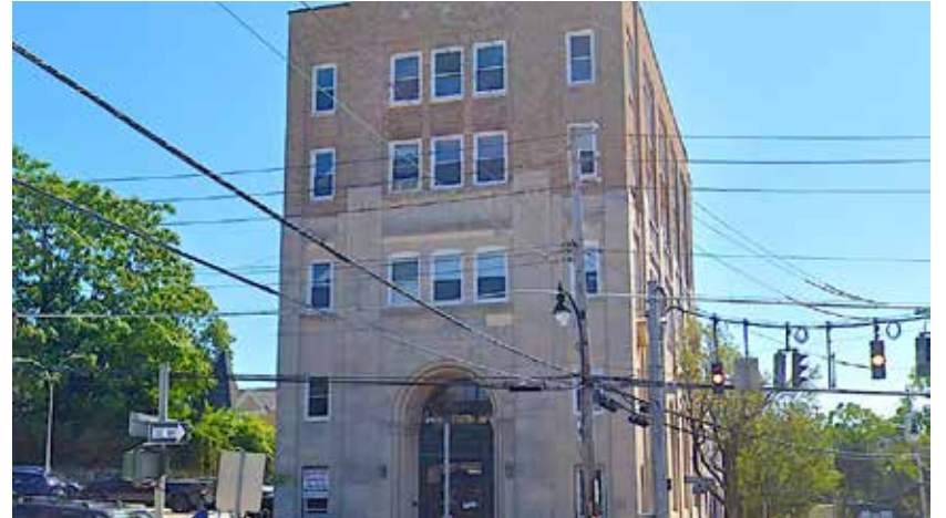
444 Bedford Road, Pleasantville. Photo via Google Maps.
