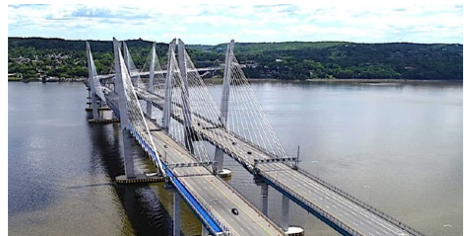
Mario M. Cuomo Bridge. Photo courtesy of NYS Thruway Authority.
