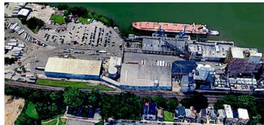
ASR refinery on Yonkers waterfront. Satellite photo via Google Maps.
