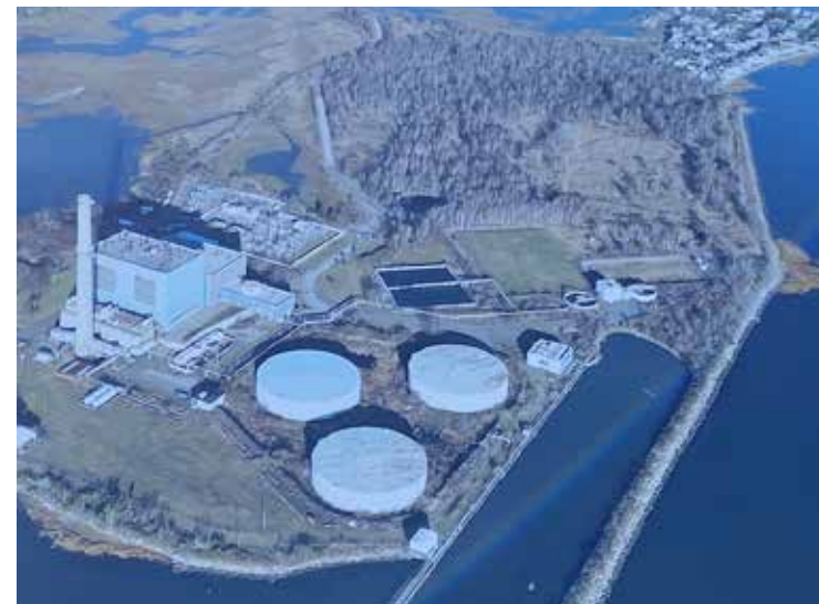
An overview photo of the oil tanks that were recently demolished. Photo courtesy of Manresa Island Corp.
