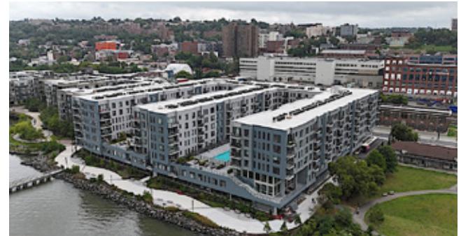
Multifamily housing development Alexander Crossing in Yonkers.
