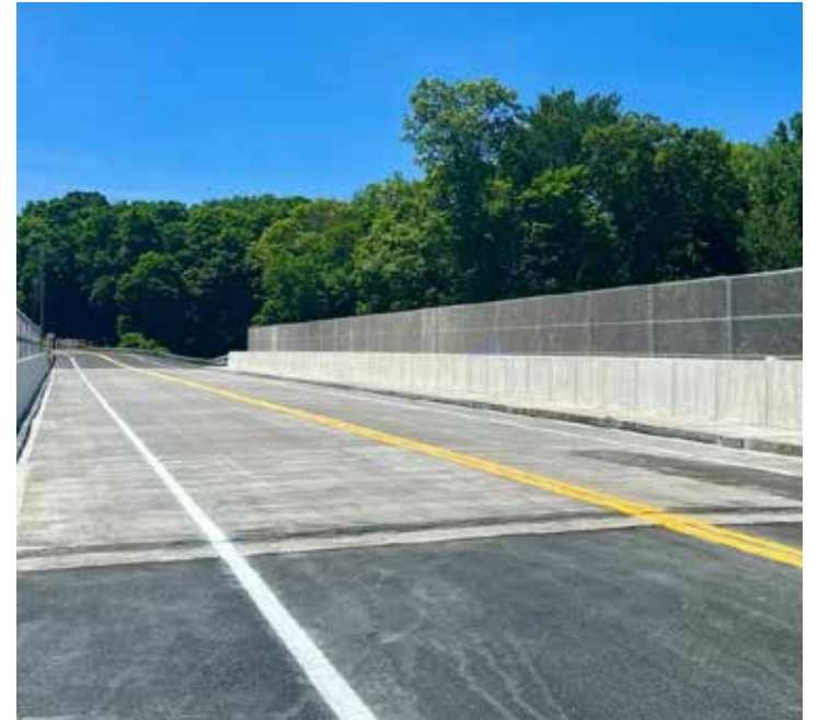
Bridge opened in Orange County Town of Newburgh.
