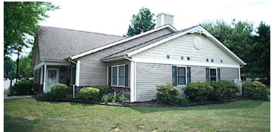
A typical building at Chambers Senior Housing.
