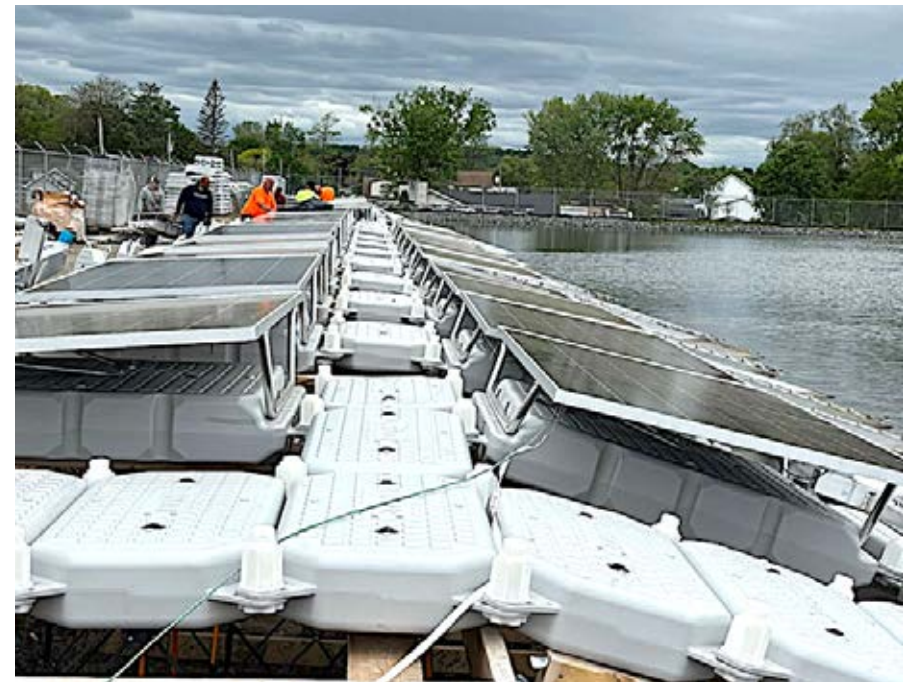
Floating solar array under construction in Cohoes, NY.
