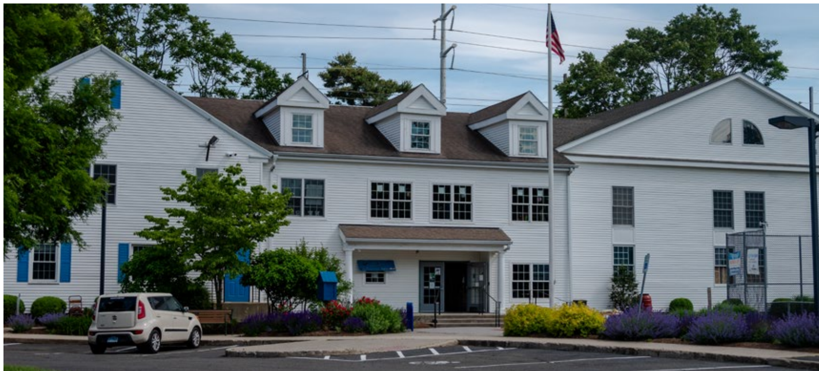
The Wakeman Boys and Girls Club is on the north side of the Metro North train tracks and could be impacted by the construction of proposed monopoles. Photo by Justin McGown.
