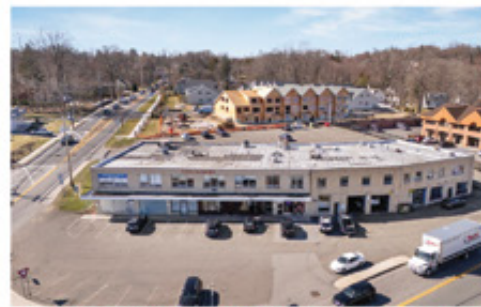
PRIME RETAIL & OFFICE BUILDING IN DOWNTOWN YORKTOWN HEIGHTS FOR SALE | Saw Mill River Rd. | Yorktown Heights, NY Listed by K. Lefkowitz & G. Klein | Call for Pricing
