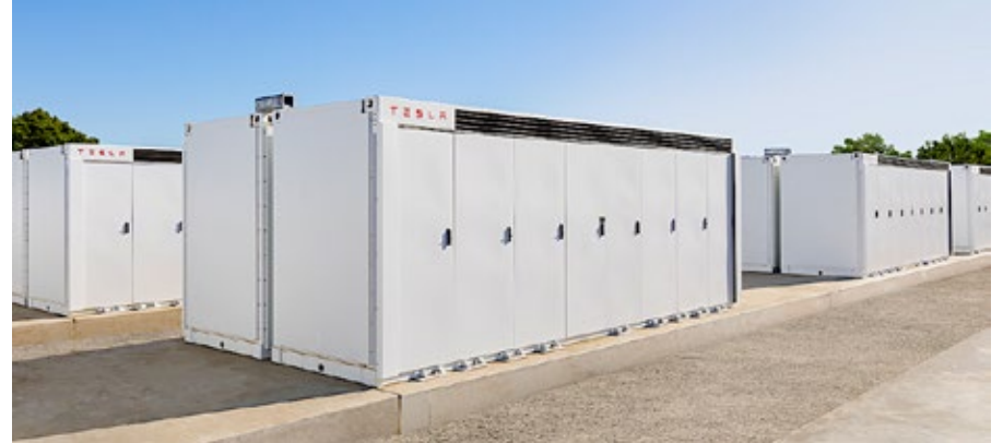
Tesla Megapack battery setup.
