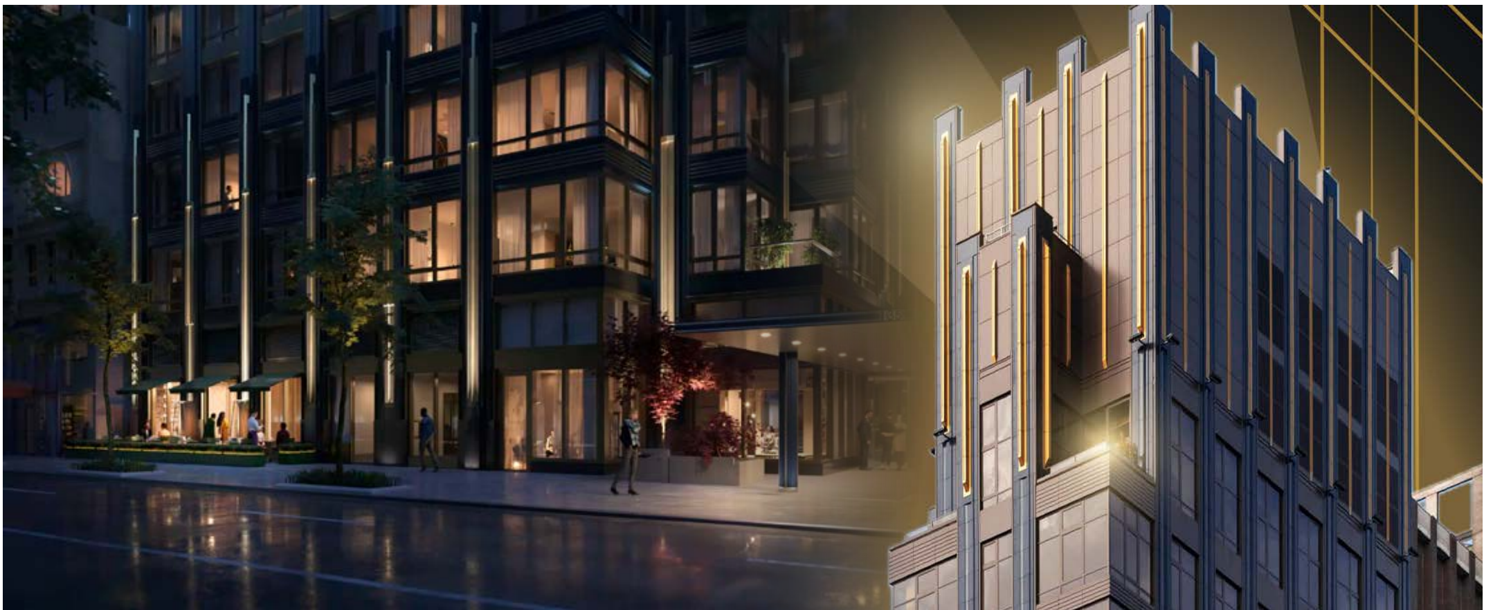
Location, location, location: The new Monogram New York nestles into midtown, a stone's throw from Grand Central Terminal. Photograph by Arch-Exist.
