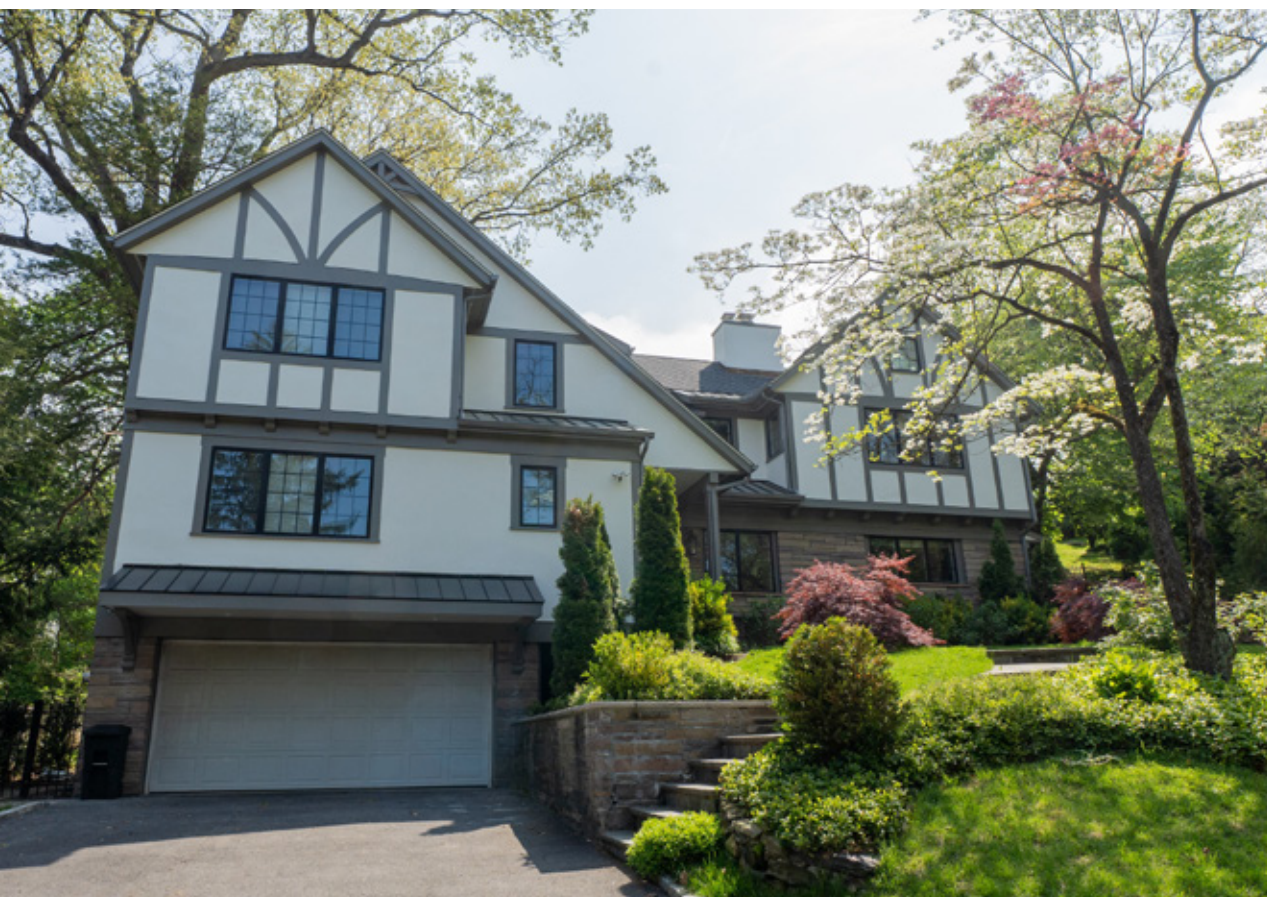
Remodeling Consultants Inc. added a full second-story addition to this Pelham Manor home. Photographs by Jorge Ulloa, Remodeling Consultants Inc.
