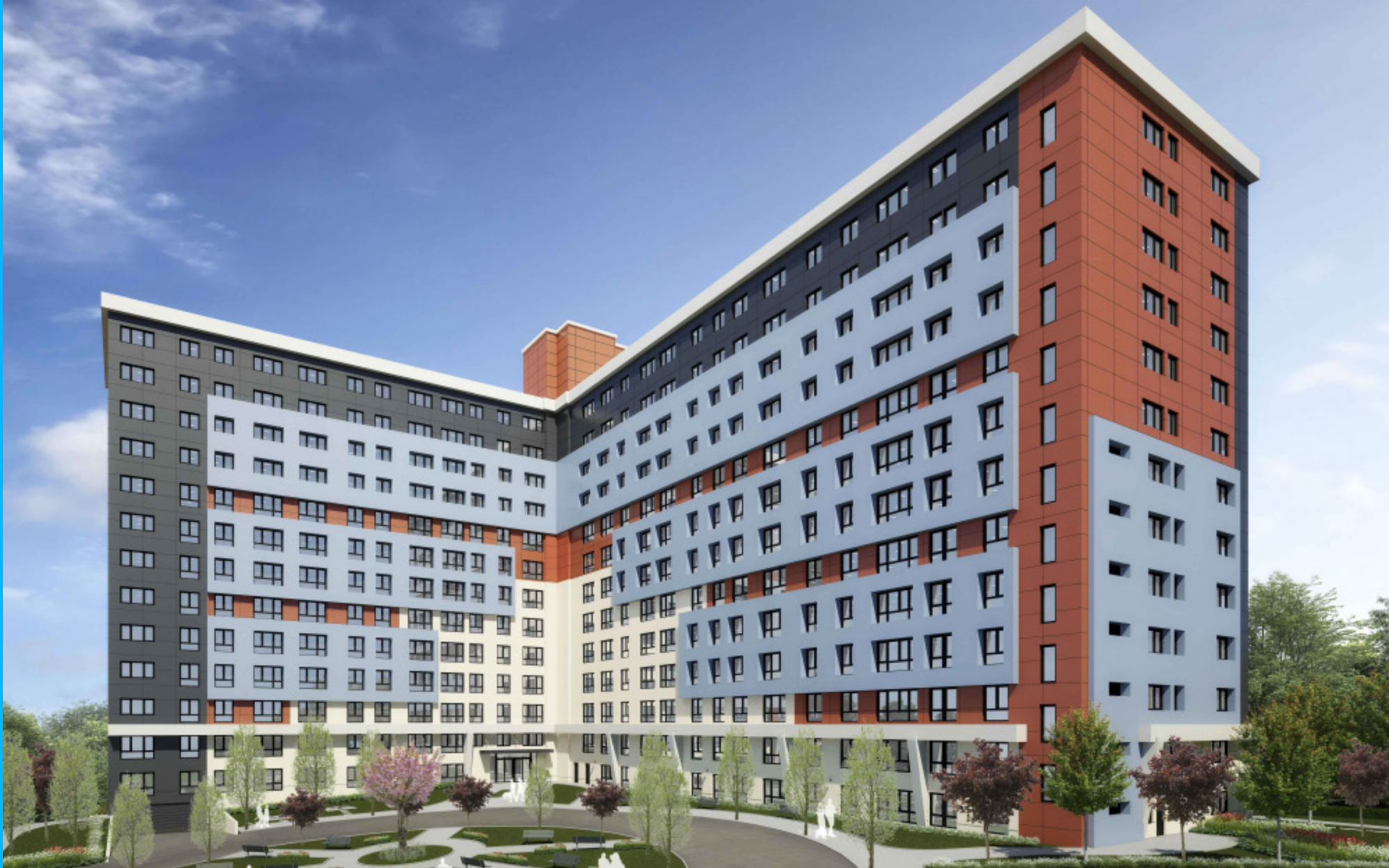
Rendering of revised building proposed for Fillmore Street and Yonkers Avenue lots.
