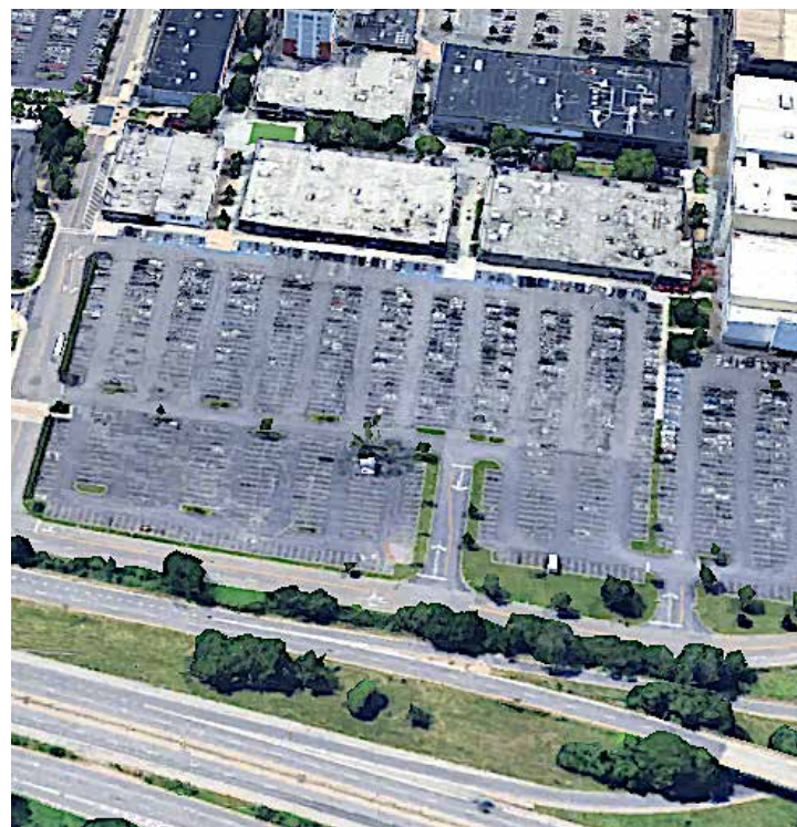
Area at Cross County Center where new construction is taking place. Satellite photo via Google Maps.
