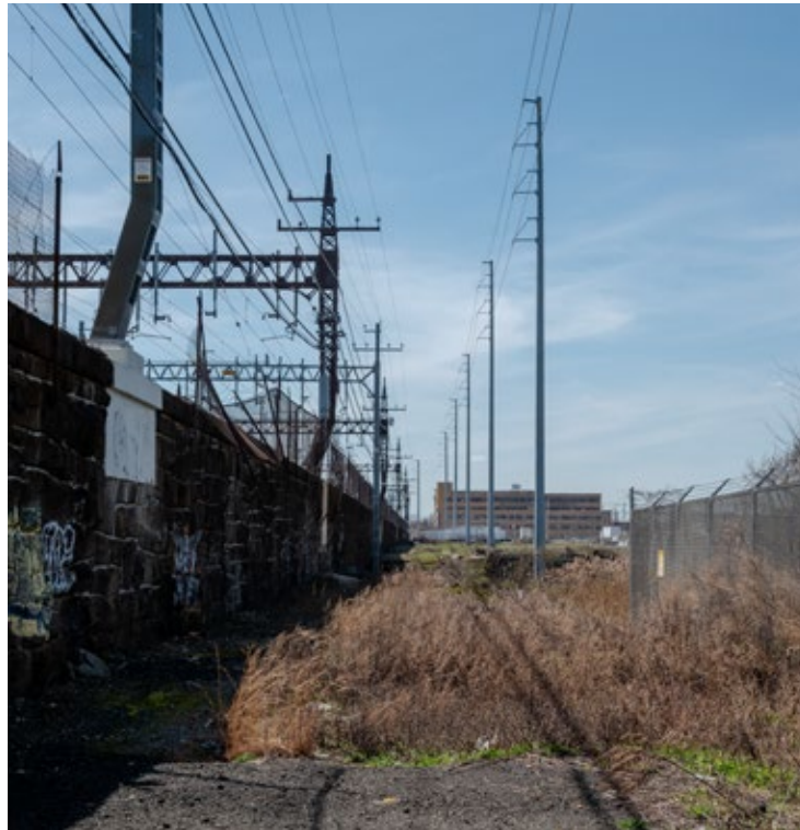
Monopoles in Bridgeport alongside a section of Metro North Railroad with catenaries. Photo by Justin McGown.
