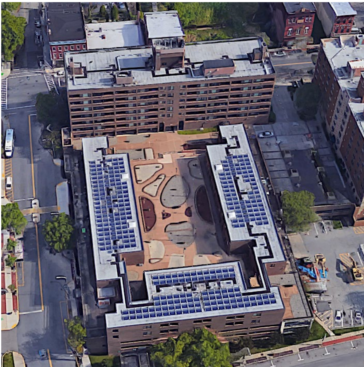
Peekskill Plaza Apartments. Satellite photo via Google Maps.
