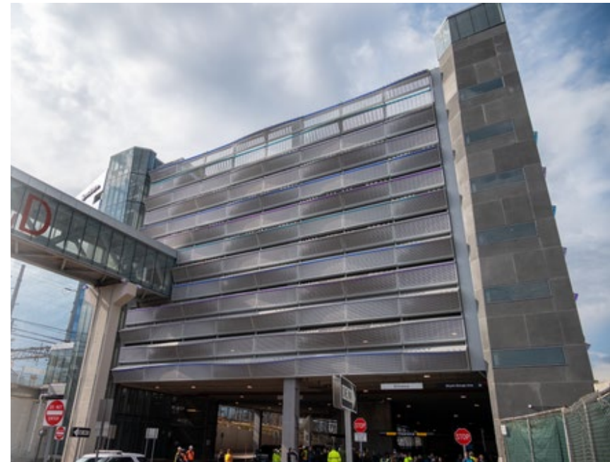
The new garage at Stamford Transit Center.
