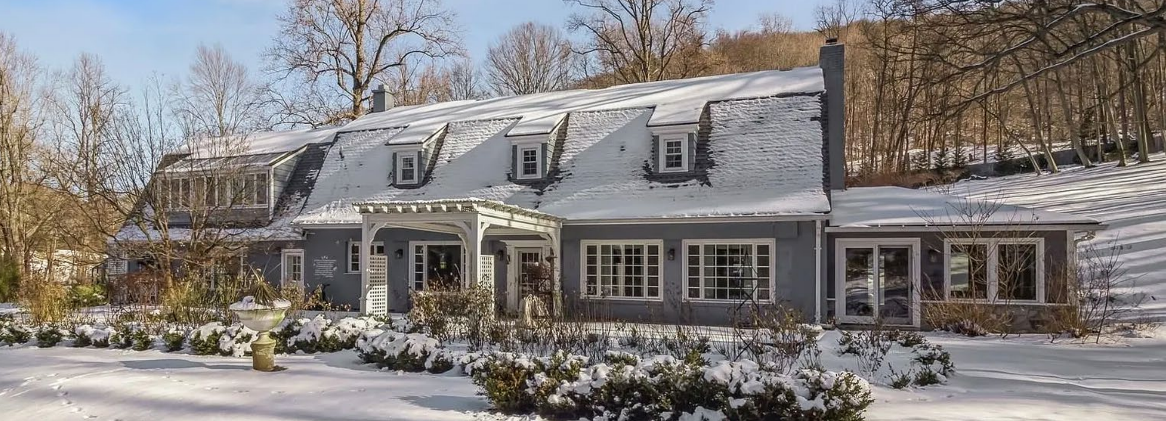
This 19th-century carriage-style house was once part of railroad magnate Samuel Sloan's Garrison estate. Photographs courtesy Houlihan Lawrence.
