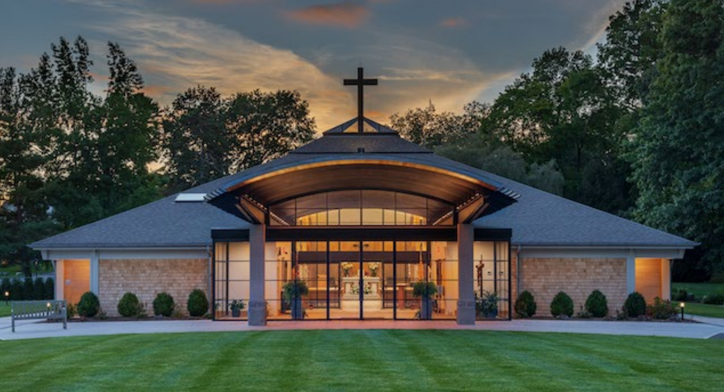
St. Michael's Church in Greenwich offers an example of a Burr Salvatore Architects renovation. Photograph by Tim Lee.
