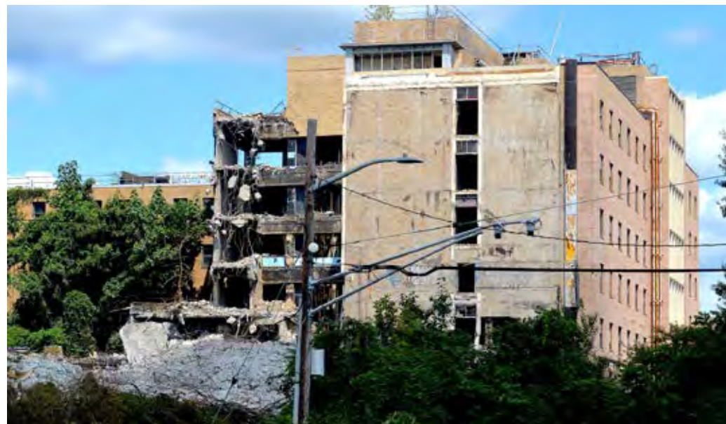
Beginnings of United Hospital demolition. Photo by Peter Katz.
