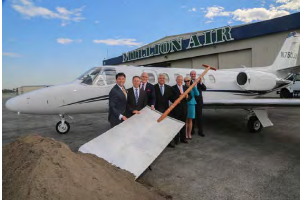
CEO Roger Woolsey; Rob Astorino; Harrison Mayor Ron Belmont; Jeff Mickler of Jacob White Construction; George Oros, chief of staff; Marsha Gordon, president of Business Council of Westchester and Deputy County Executive Kevin Plunkett at Million Air's groundbreaking at Westchester County Airport.
