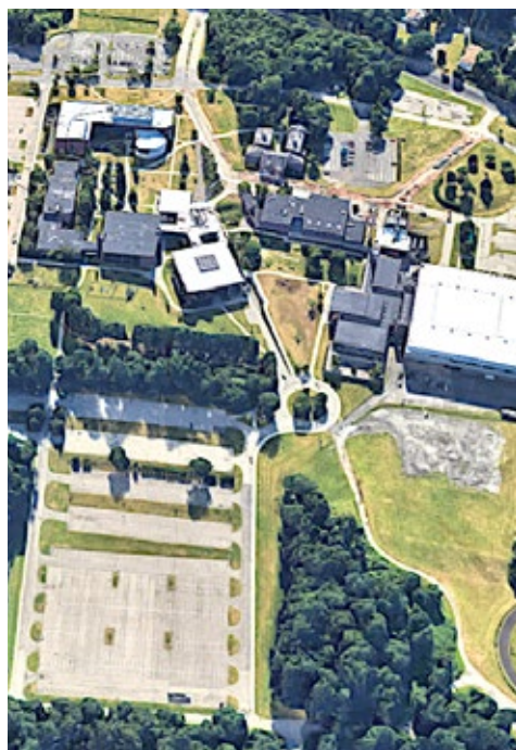
Rockland Community College. Satellite photo via Google Maps.
