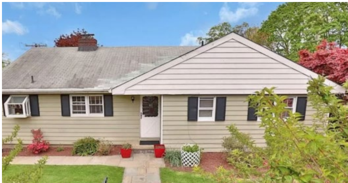
Ossining home improvement project
