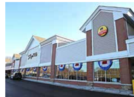
Exterior of the new Elmsford-Greenburgh ShopRite.
