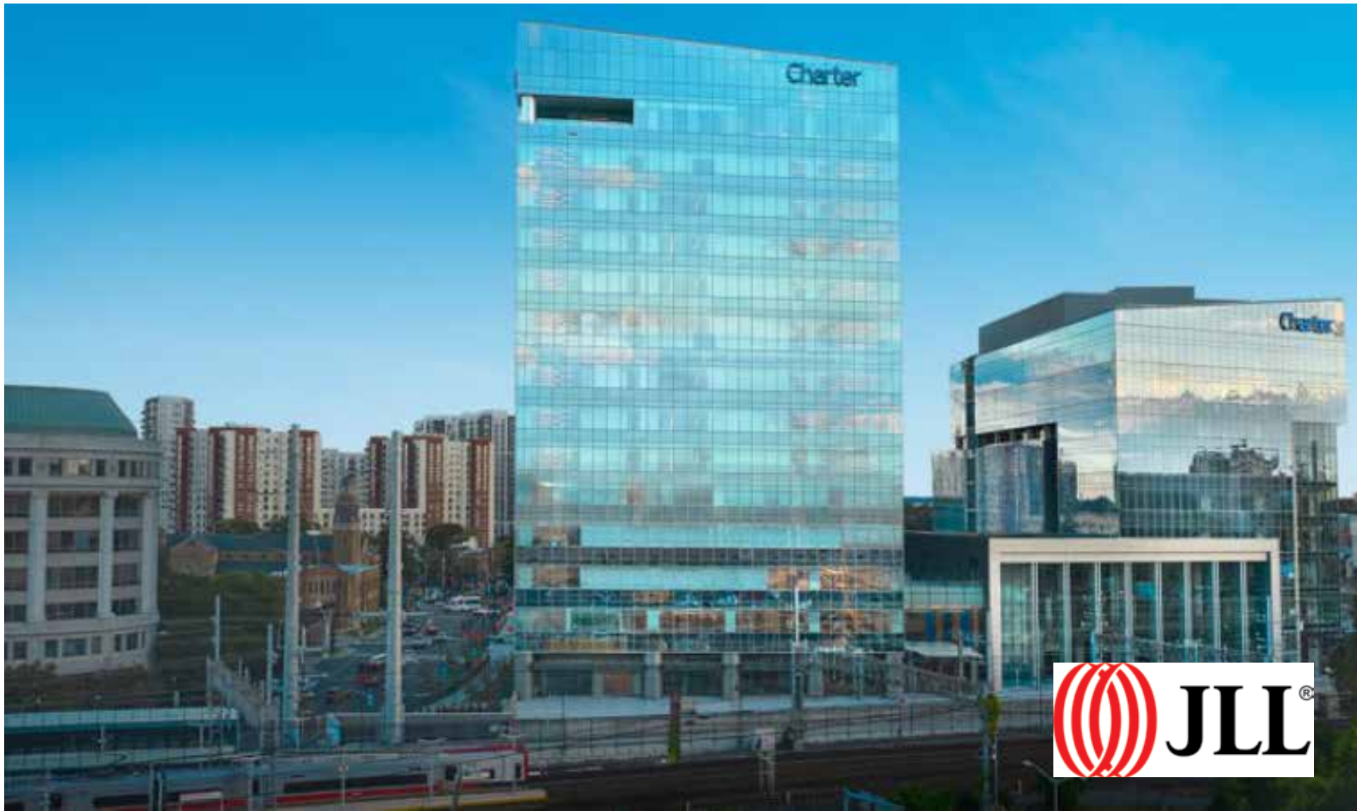
Charter Communications HQ in Stamford, CT.
