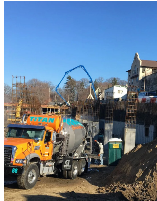
Titan Concrete on the job
