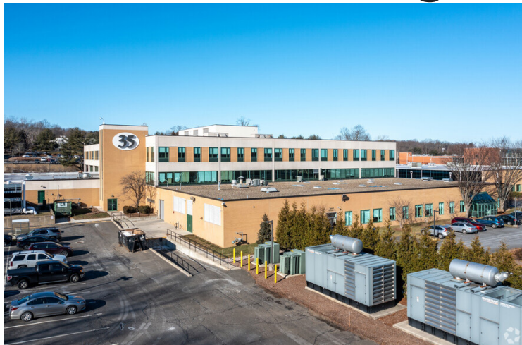
35 Nutmeg Drive in Trumbull. Photo courtesy of LoopNet.
