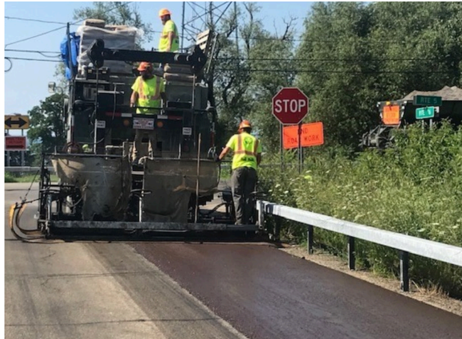
Repaving a local road. NYS Department of Transportation photo.
