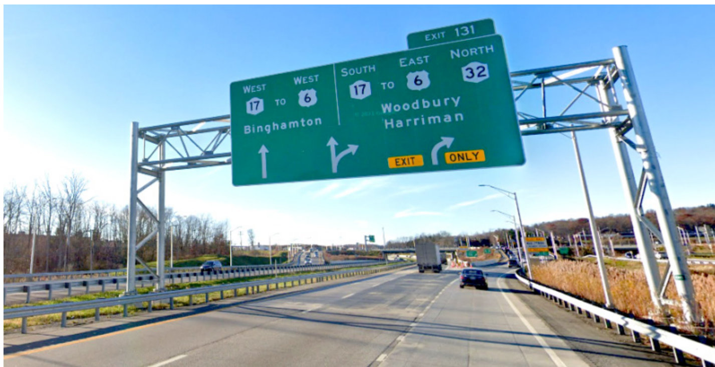
Route 17 near Woodbury Common. Photo via Google Maps.
