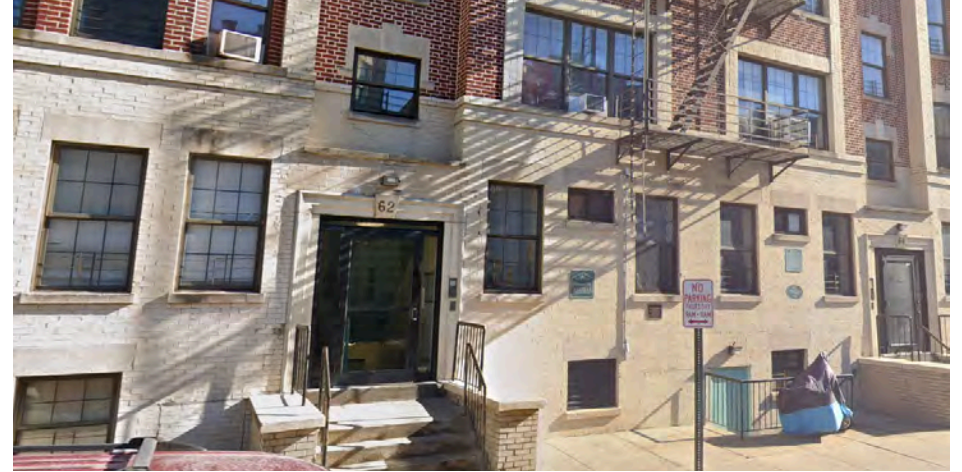
Westhab apartments, Elliot Avenue, Yonkers.
