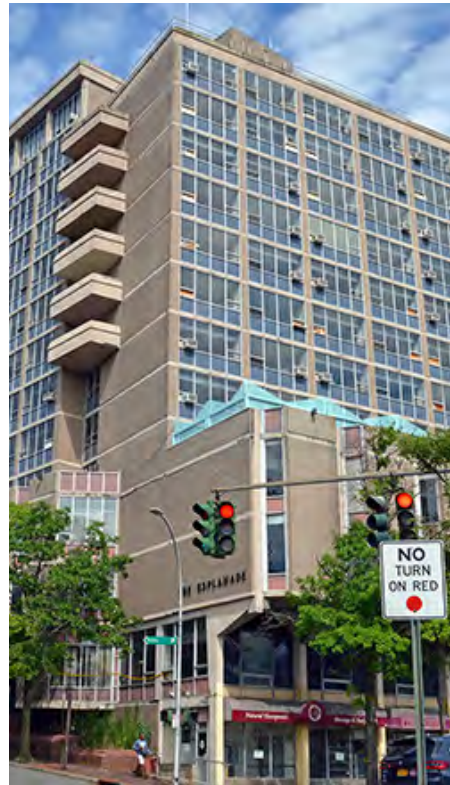
The former Esplanade in White Plains. Photo by Peter Katz.
