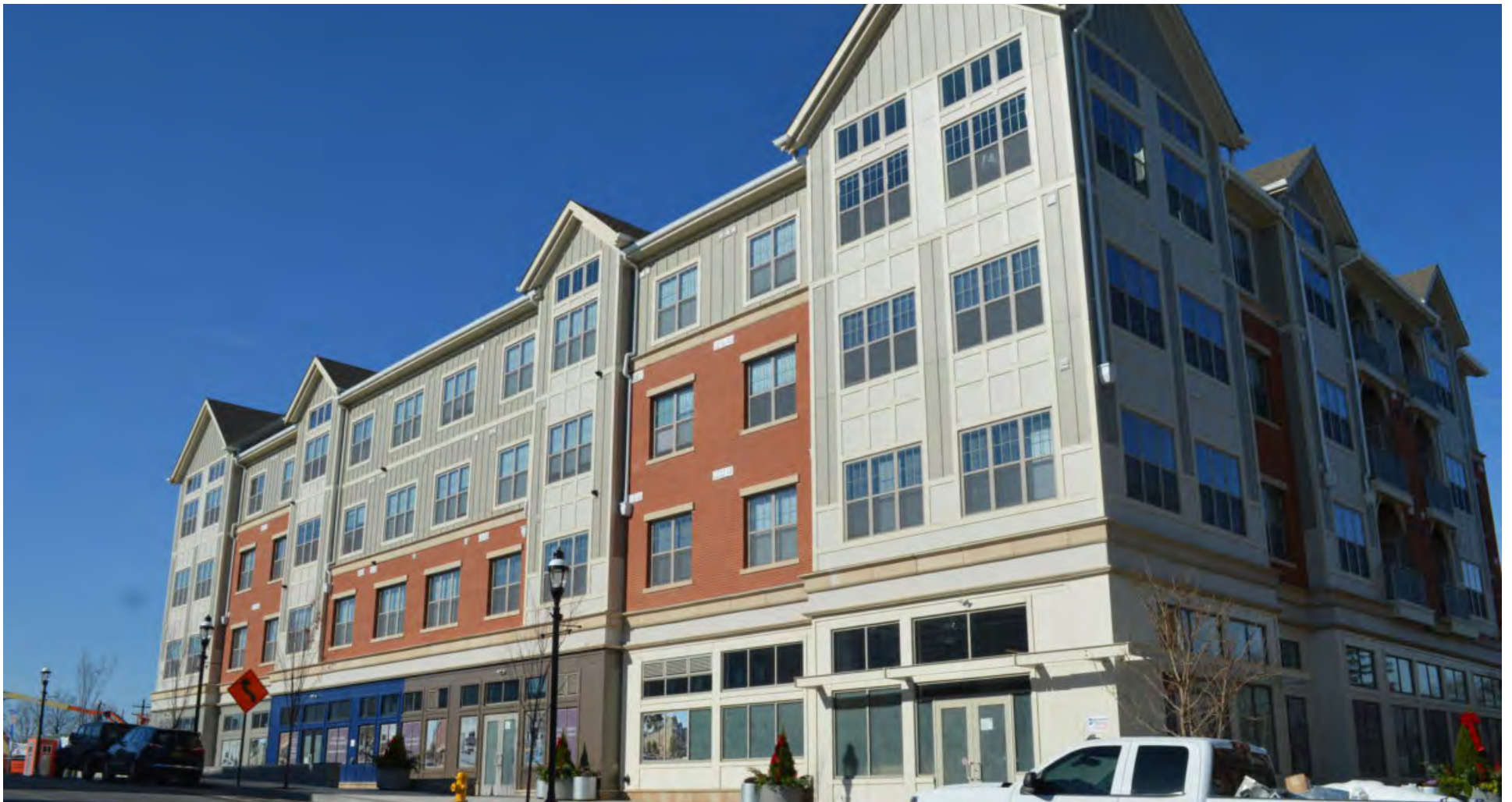
Avalon Bay project at Harrison train station on Nov. 21, 2021. Photo by Peter Katz.
